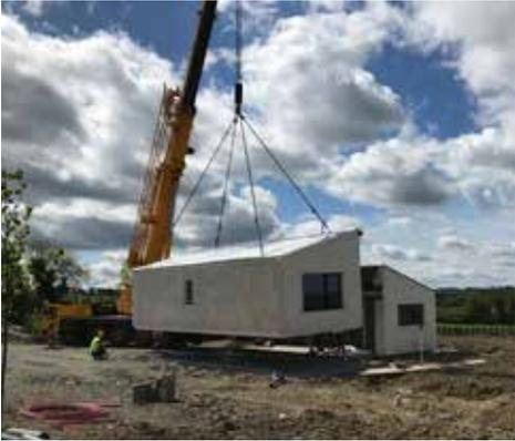
Now that the modules are finished and the site is prepared, things really start to speed up! Our installation team will arrive on site early that morning, set up the crane and begin lifting the units into place. Finishing up the junction details internally and externally as well as connection of services will typically begin on day 2.
